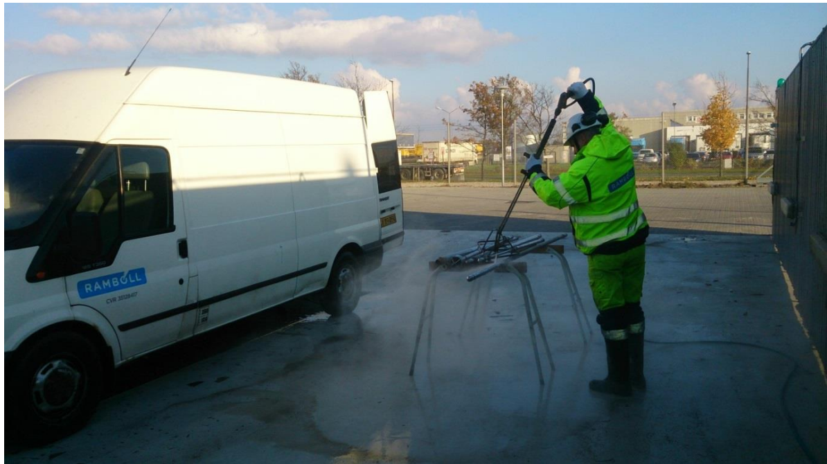
Figure 2-1: High pressure cleaning of logging tools.
